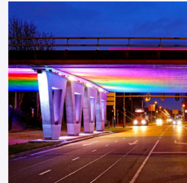
Light art under the bridge as an entrance gate to the area.
